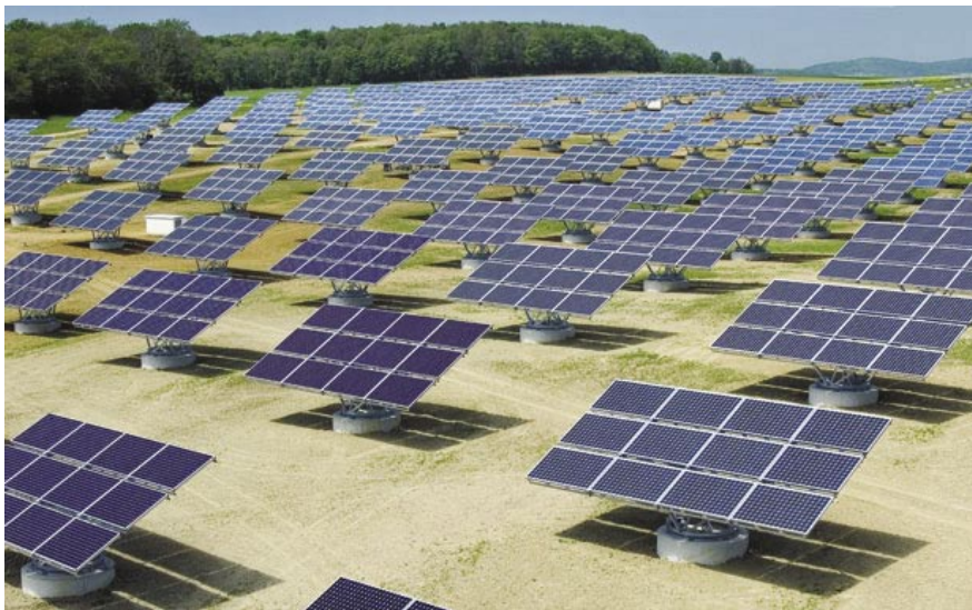
Figure 1. Solar parks are rapidly becoming the norm in Germany, where a single solar tracking installation that follows the sun across the sky can be as large as 117 football fields. This one is at Gut Erlasee. Photo: Paul Langrock
